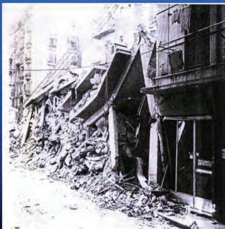
Fig. 5 Apartment building in Ippodromiou Sq., Thessaloniki. View taken from point A (Fig. 1) at Nikiforou Foka Str., 30 hours after collapse.
