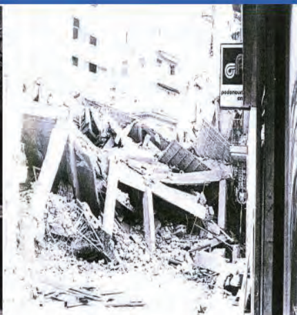
Fig. 6 Apartment building in Ippodromiou Sq., Thessaloniki. View taken from point I (Fig. 1) at George Theotari Str., 30 hours after collapse.
