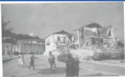
Figure 13 - Collapse of old masonry houses in Kalamata.
