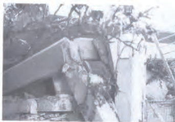
Figure 20 - Close-up view of the collapsed building of Fig. 19, showing poor joint construction.
