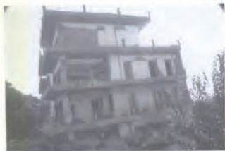
Figure 17 - Apartment building on pilotis. The pilotis (ground) and the first story collapsed while the rest tilted dangerously.
